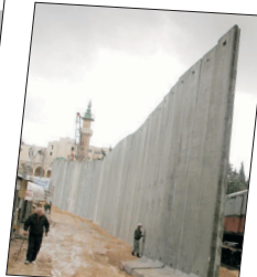
The walled portion of the barrier is 32-35 feet high. In E. Jerusalem cuts through Palestinian neighborhoods.
